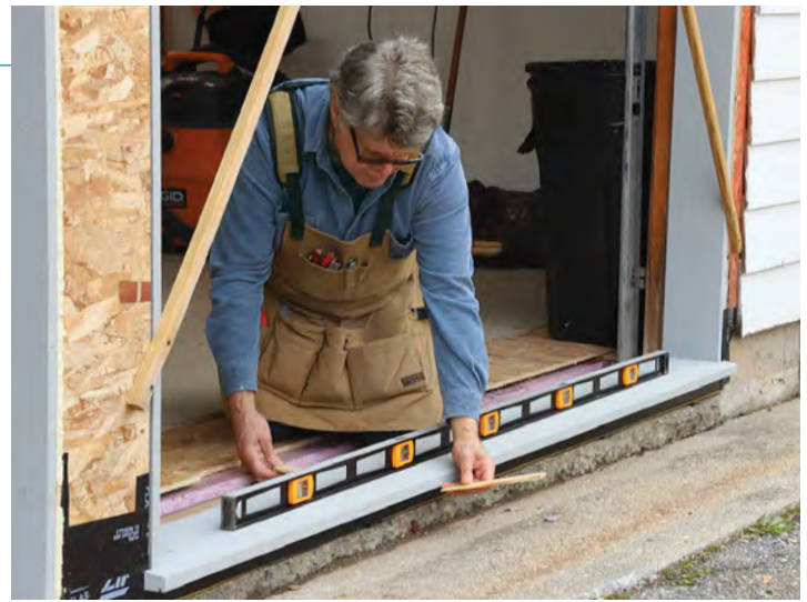
Level the threshold. With the jambs in place, level the threshold, adding shims where necessary.
