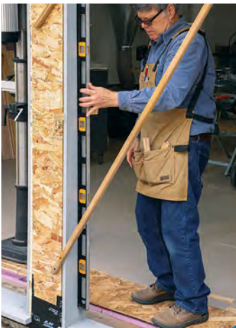
Plumb the jamb. Once the threshold is level, check that the side jambs are plumb and straight. Add shims where needed.
